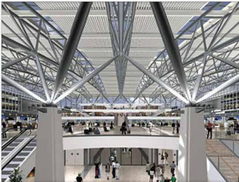
Figure 17: Building with Tubular Structures, Column Trees and "Banana" Trusses, Source: Civil.IITB
