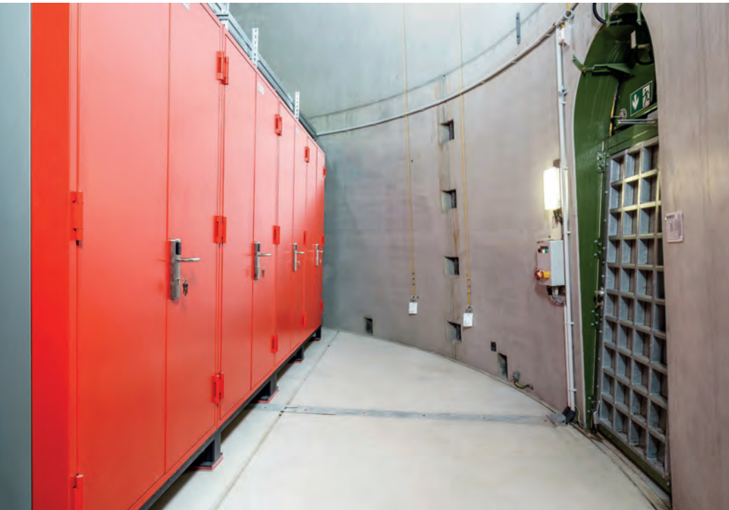
Figure 1: View inside the tower of the wind turbine
