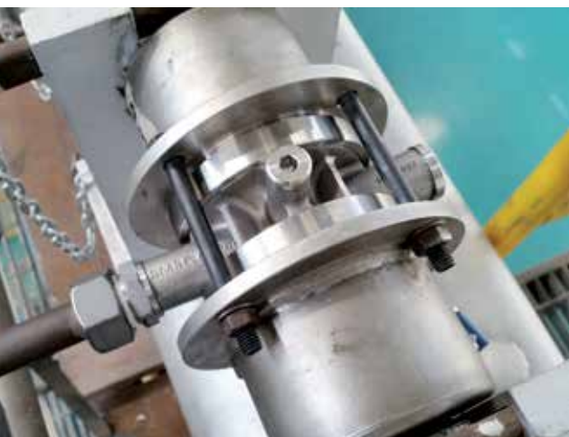
Installation of the nozzle at BIRLA COPPER
