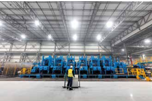
Shaping section, 28-inch ERW tube welding line at Zekelman Industries, Blytheville, USA
